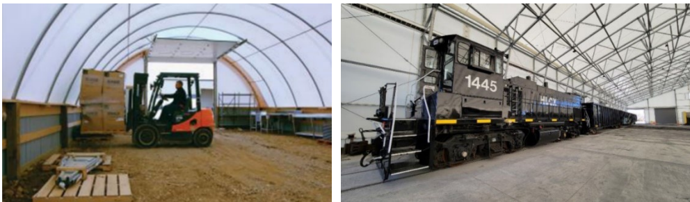
Figure 3: On the left an example of Single Truss building style, photo courtesy of Norseman Group Ltd. On the right an example of Double Truss building style, photo courtesy of GNB Global.
