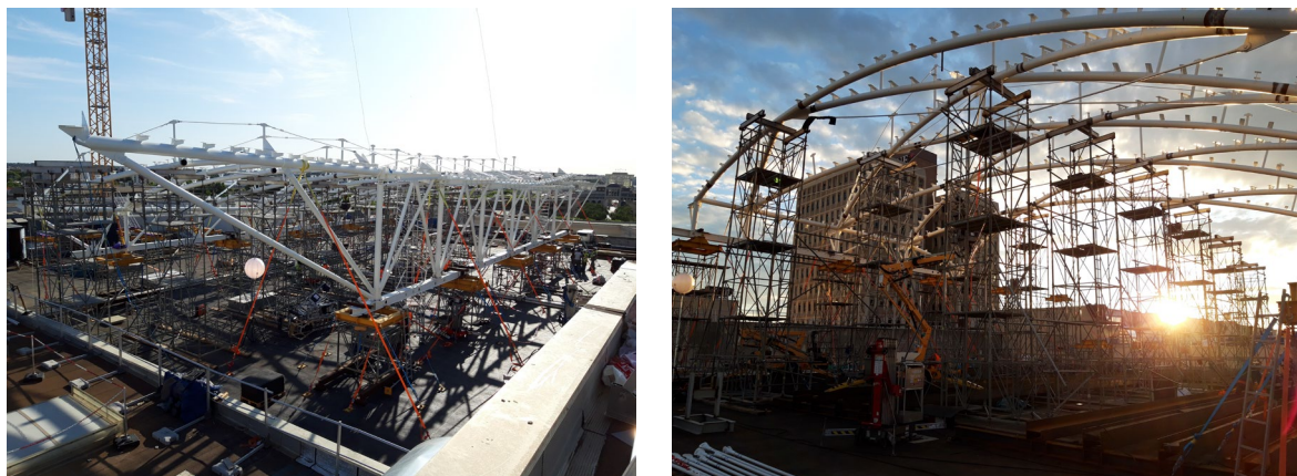
Figure 4: Assembly of the metal structure on the adjacent working platform.
