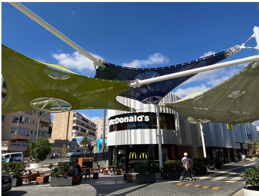
Figure 5 Porto Pi drive through entrance's pergolas
