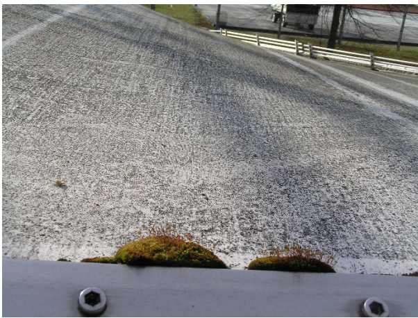
Figure 2a: PTFE/Glass fabric after 11 years
