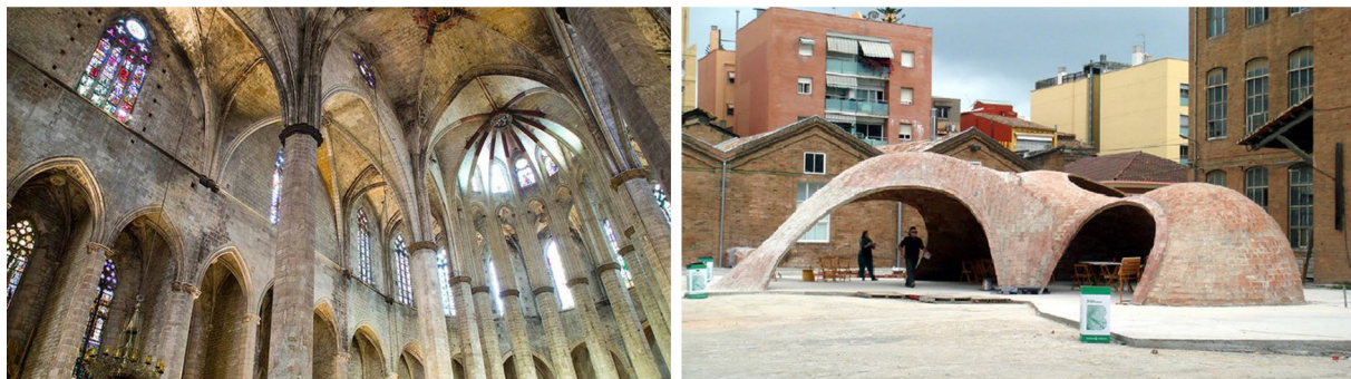
Figure 4 Santa Maria del Mar, Barcelona (1329-1383): gothic structures direct loads through lines. Figure 5 Brick-Topia, Fabra i Coats, Barcelona, 2013: a thin only compressed ceramic vault.
