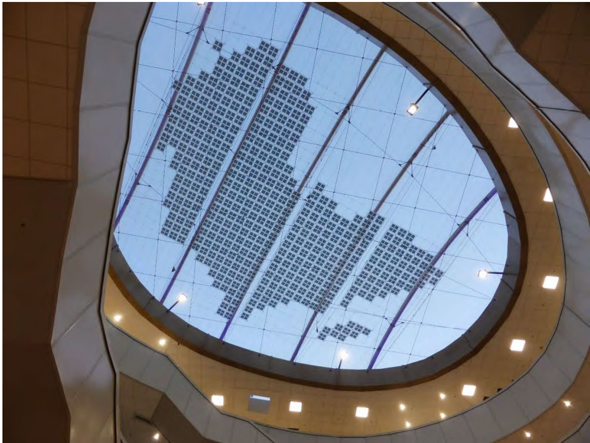
Figure 10: ETFE cushion atrium roof including photovoltaic modules
