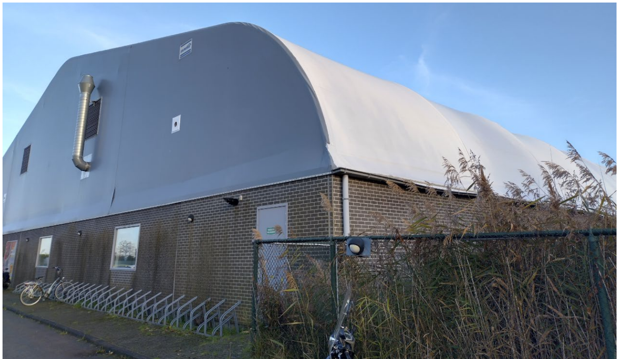
Figure 1: External view of a PE / PE membrane for an indoor tennis court
