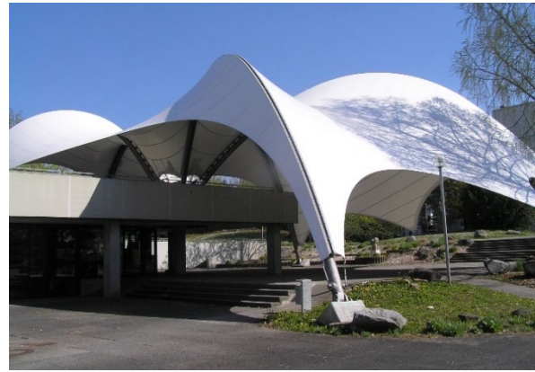
Figure 5b: Situation today with vandalism in 2016 on the left side
