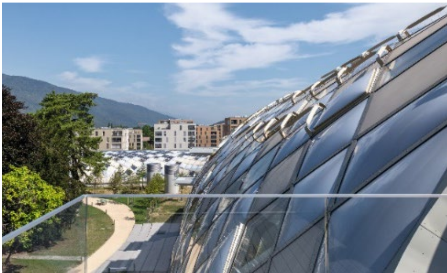
Figure 2: Exterior view from a balcony, ©Swatch Omega AG
