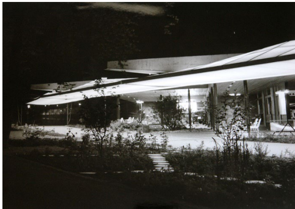
Figure 4a: Textile canopy entrance building spa garden Bad Wildbad, Germany 1964, Archive Bauamt Pforzheim
