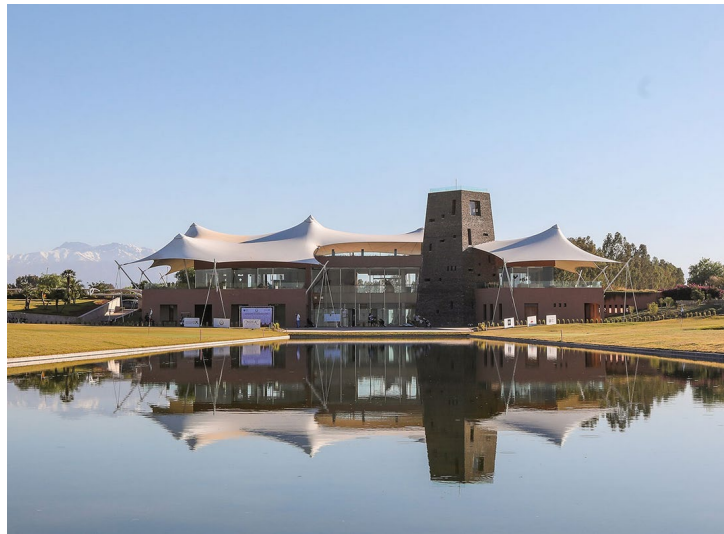
Figure 1: External view of the micro climatic roof: Chrifia golf club house – Morocco Architect: Youssef Melehi, Rabat – Morocco / Engineering: Prat SA – France / Membrane fabrication & installation: Ametema – Morocco / Membrane: Serge ferrari Flexlight 1202 S2 – 1500 sqm
