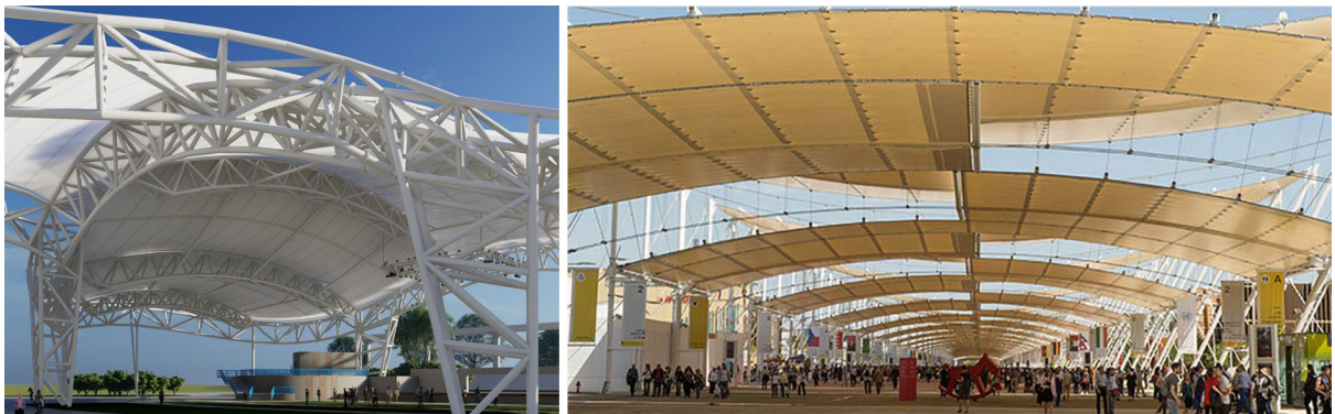
Figure 10: Imagine Clearwater Amphitheater, 2022: the membrane rests on the steel structure. Figure 11: Cardo e Decumano streets, Expo Milano 2015. The membrane hangs from cables. The primary structure is reduced to the lateral masts. Bending is avoided.
