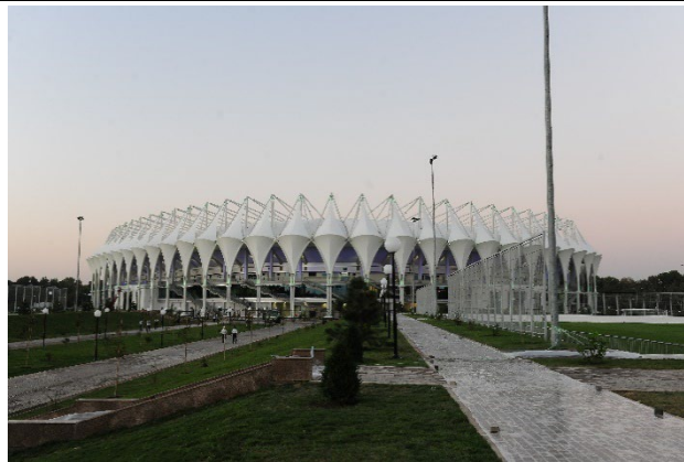
Figure 1: Tashkent Stadium, SATTLER GROUP
