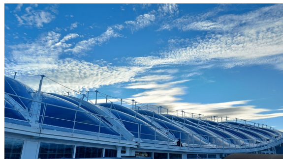
Figure 2: On the left, increased natural light through the new ETFE cushion cover; on the right, external appearance of the constantly variable roof geometry.
