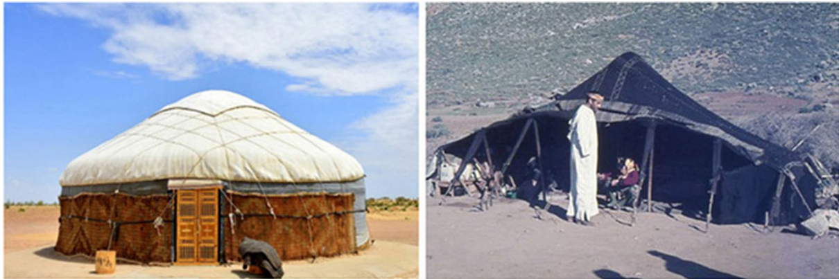
Figure 8: The yurt is supported by a lattice of wood. Figure 9: the jaima tent is properly a structural membrane. Both illustrate that de dilemma is as old as mankind.
