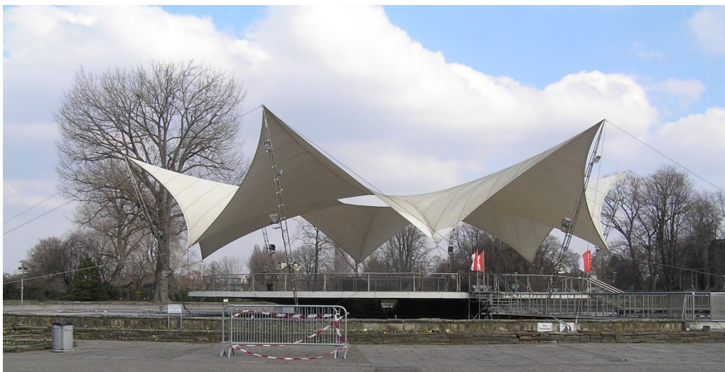
Figure 6: Tanzbrunnen Köln, 3 times replacement of the fabric, one-time replacement of the cables, build 1957, picture 2016
