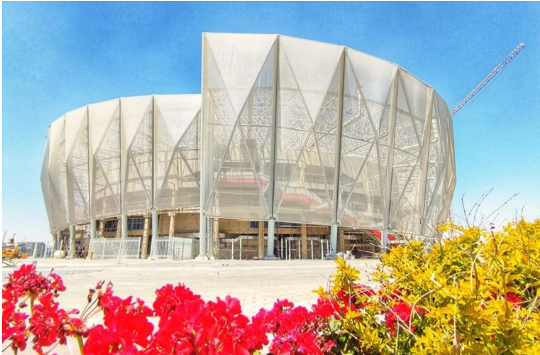
Figure 14: The final look of the facade with the perforated fabric and the visible structure behind
