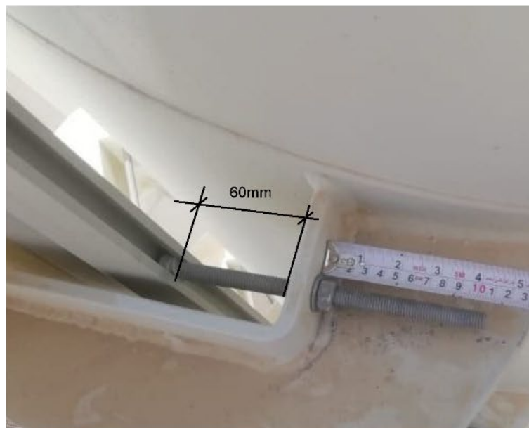
Figure 6: Facade tensioning system which ensures the long-term functioning of the facade system
