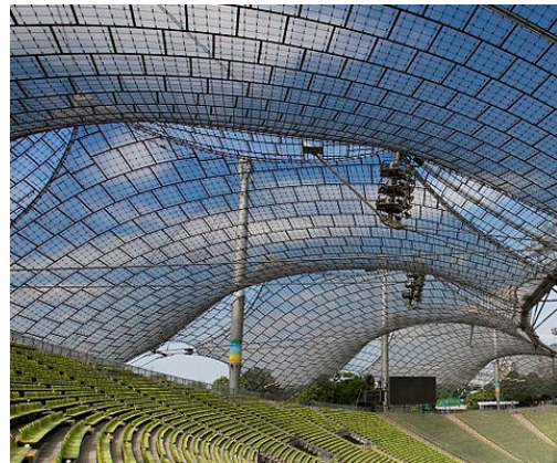
Figure 12: Olympic Stadium in München, structural design Frei Otto, Wikimedia-licenced © Jorge Royan
